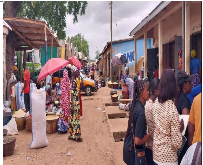
Uncovered drains pose a danger to market users
